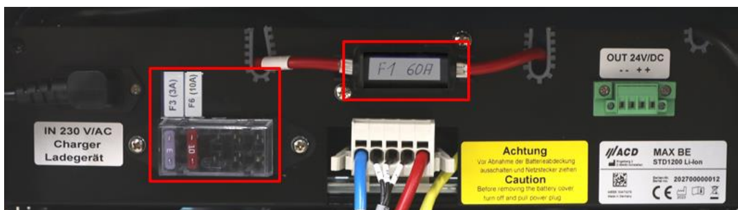
Figure 33: MAX BE 750/1200 Li-Ion and MAX Plus 750/1200 Li-Ion fuses
