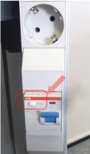
Figure 4: Test button of the residual current circuit breaker (RCD)
